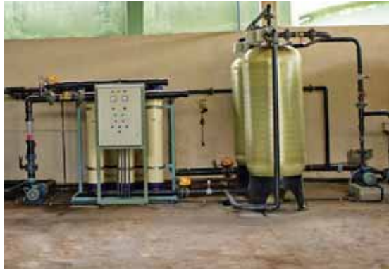
The UF plant further filters the effluent, to purify the content
